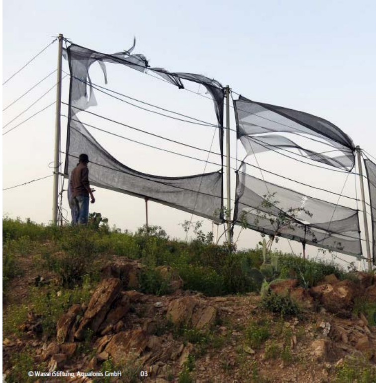
Figure 15: Preliminary net designs failed because they couldn't withstand wind speeds in the area (Aqualonis, 2015)
