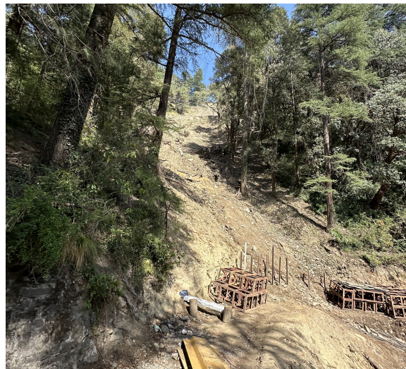
Figure 18: Aftermath of the 2023 Shiv Bawdi temple landslide in Shimla.
