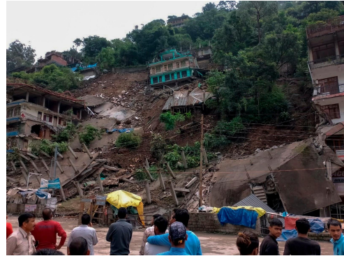
Figure 1: Landslide in Kullu, Himachal Pradesh (AP, n.d.)
