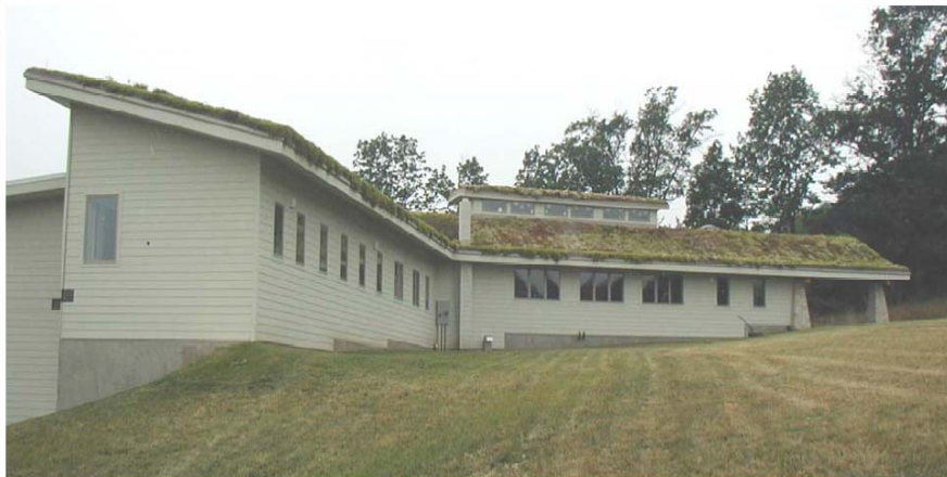
A building with an extensive green roof installed (Wark, 2003).
