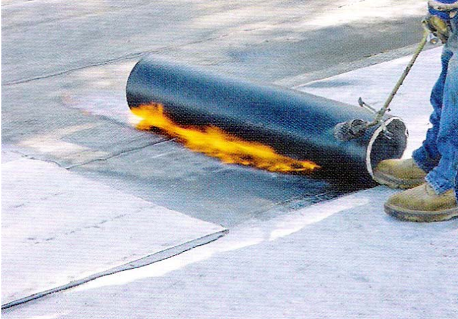
Figure 6 Heat Welding
