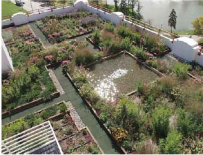
Figure 11 Implementation of an intensive green roof
