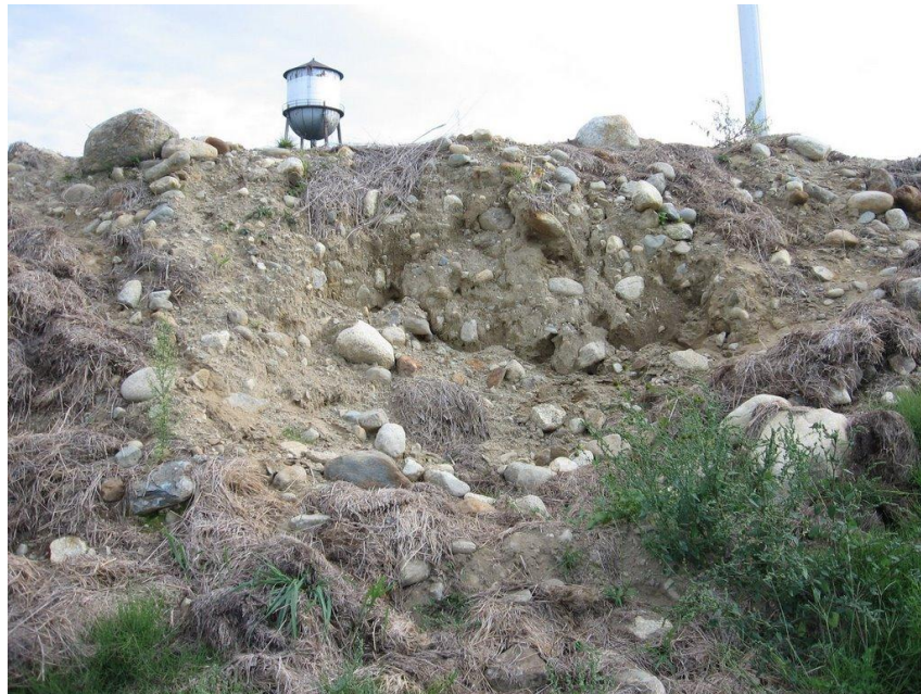
Figure 8 - View of the existing left embankment.
