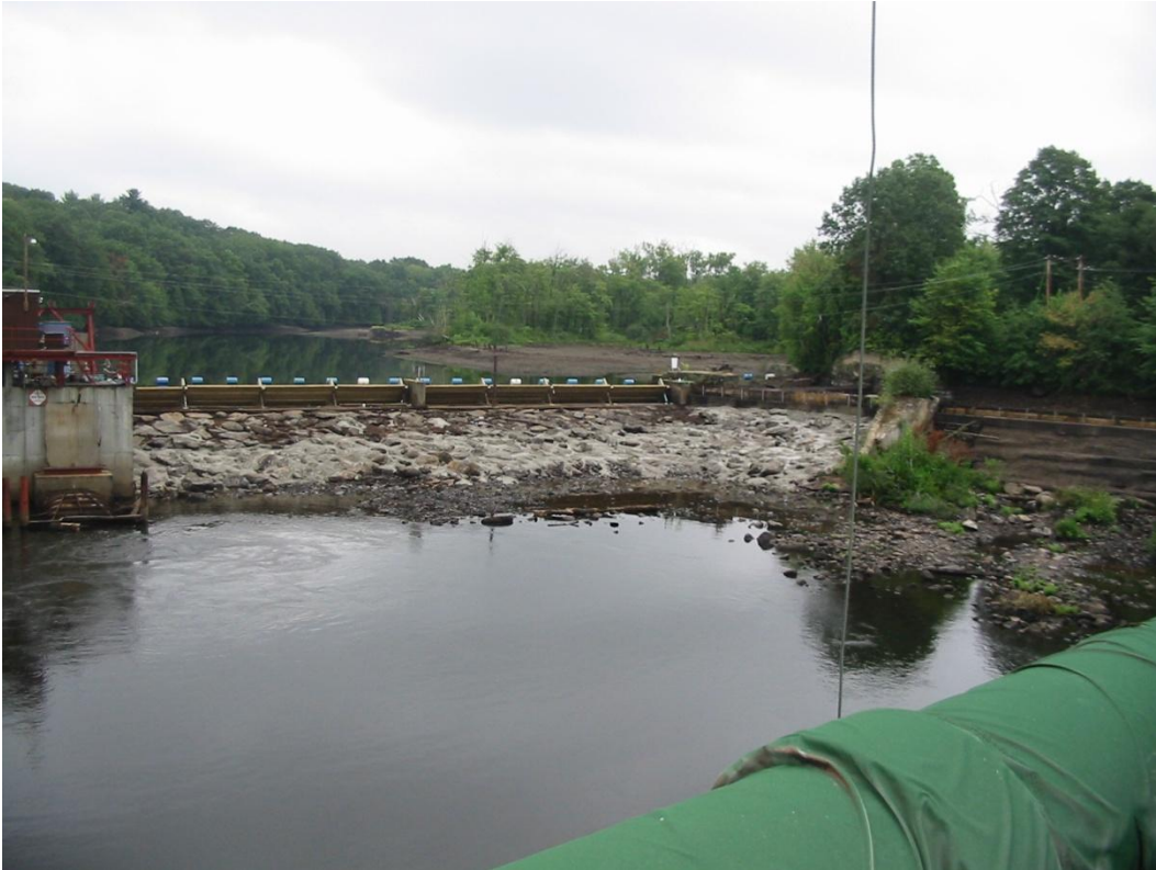
Figure Six: Summer of 2006 rehabilitation. Note all the wooden panels have been replaced. The blue barrels in the background are the boater safety buoys.
