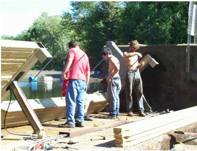
Figure 39 – The crest gate dam is visible because of repairs. (Wilbraham, Ma)
