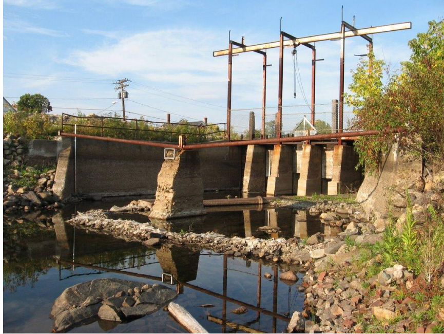
Figure 3 - Upstream of existing spillway.
