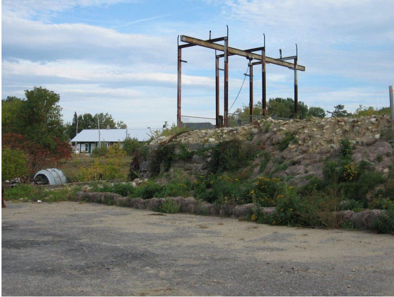
Figure 5– Existing left embankment.
