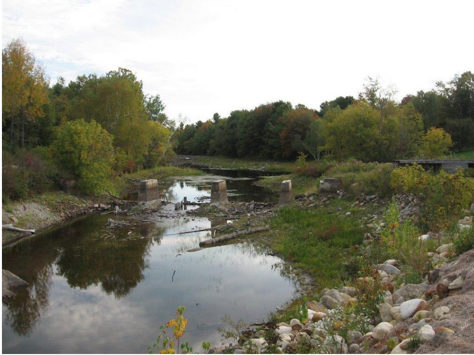
Figure 9 – View upstream of spillway including the abandoned bridge foundation piers.
