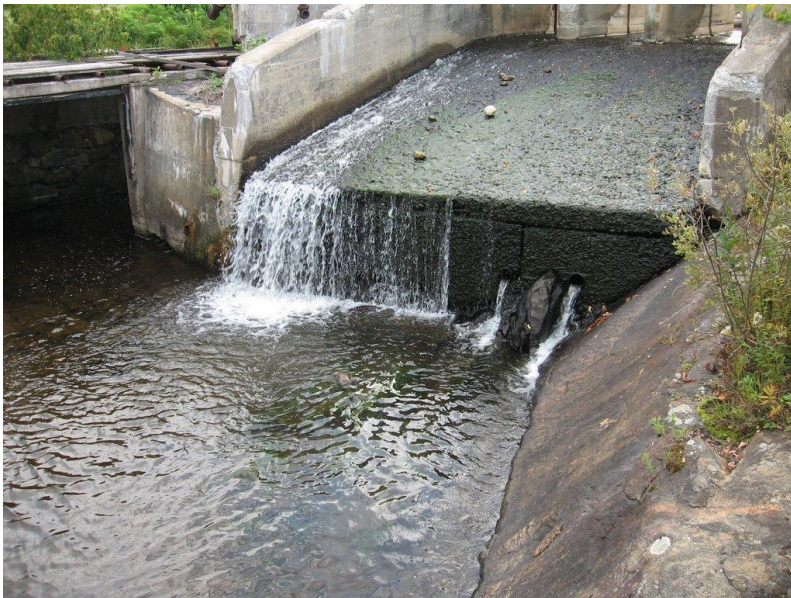
Figure 6 – Looking upstream at the existing spillway.
