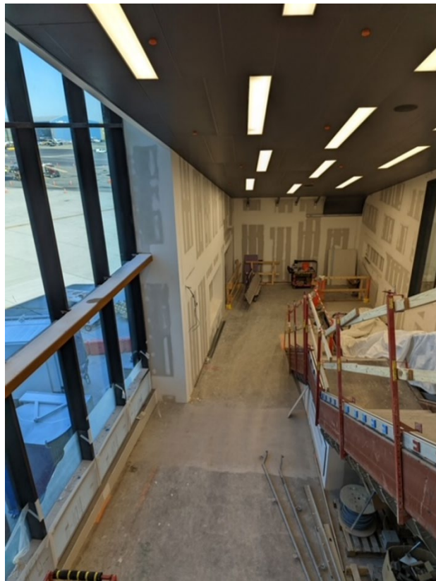
Figure 2.14: Photo of Passenger Boarding Bay from Renovation Crescent
