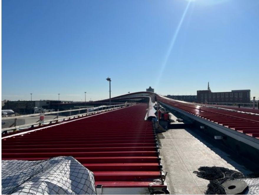
Figure 2.3: Photo of the Roof Taken from the Team's Site Visit
