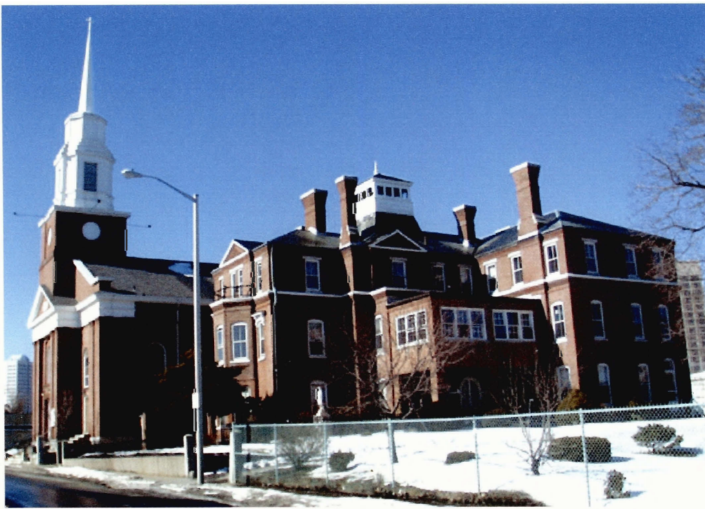
Figure 2: Saint John's Church and Rectory
