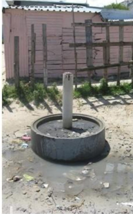
Figure 10: Standing Water at a Water Tap in C Section (Granfone et al. , 2008)
