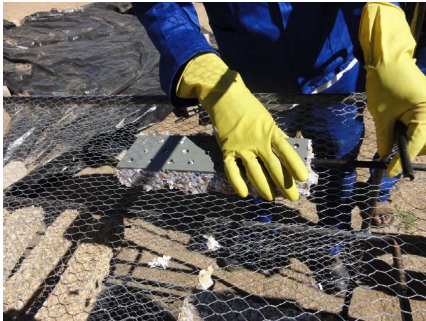
Figure 59: Pulling rods out of block
