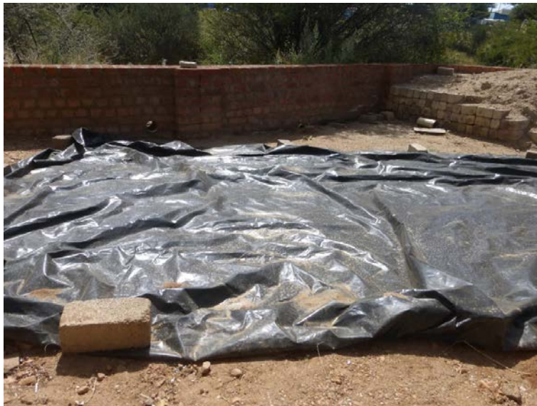
Figure 44: Large black tarp for drying blocks
