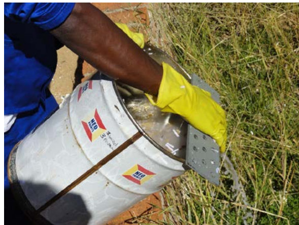
Figure 48: Removing excess water from mixture
