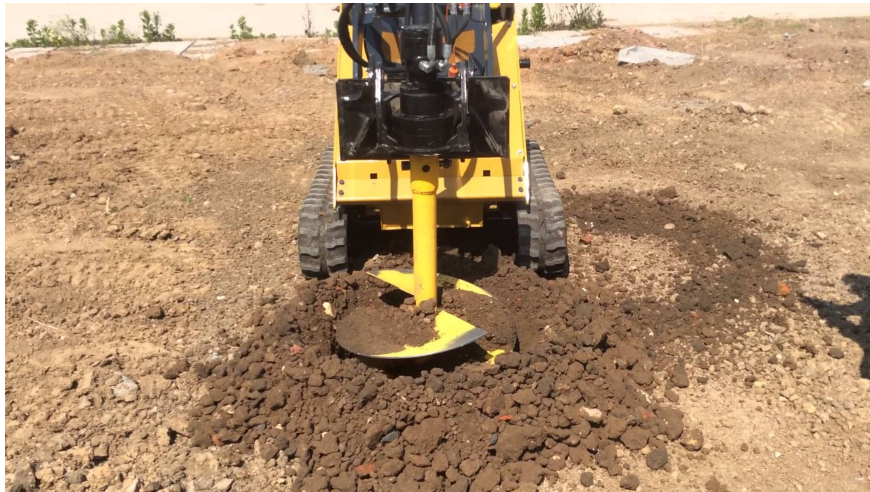
Figure 6: An Auger Drill in Action 8 .
