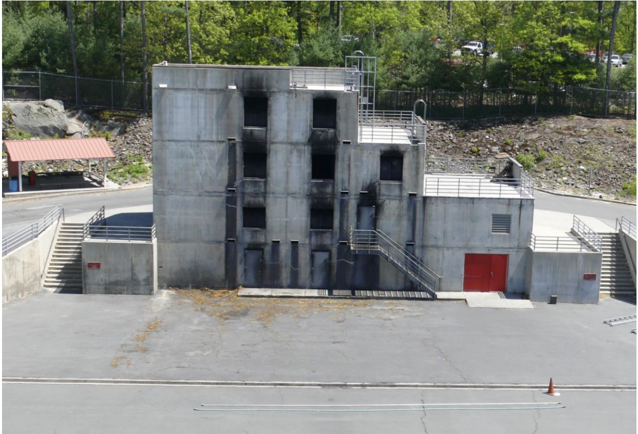
Figure 29: Image of MA Firefighting Academy Burn Building (MAFA, 2021)
