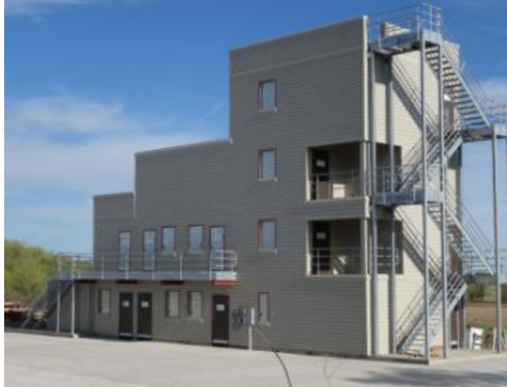
Figure 3: Elaborate Fire Training Tower (Fire Facilities Staff, 2020)
