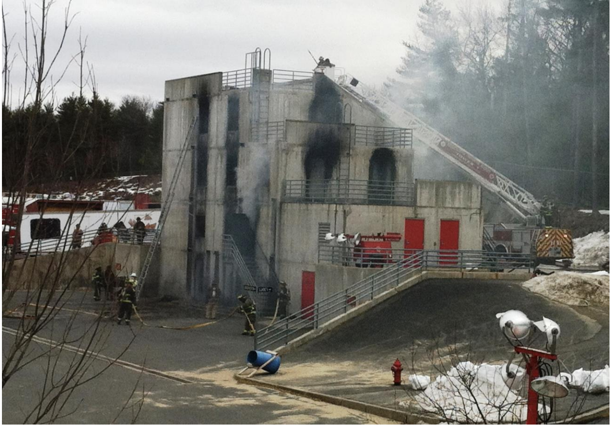
Figure 30: MA Firefighting Academy Burn Building in Use (MAFA, 2021)
