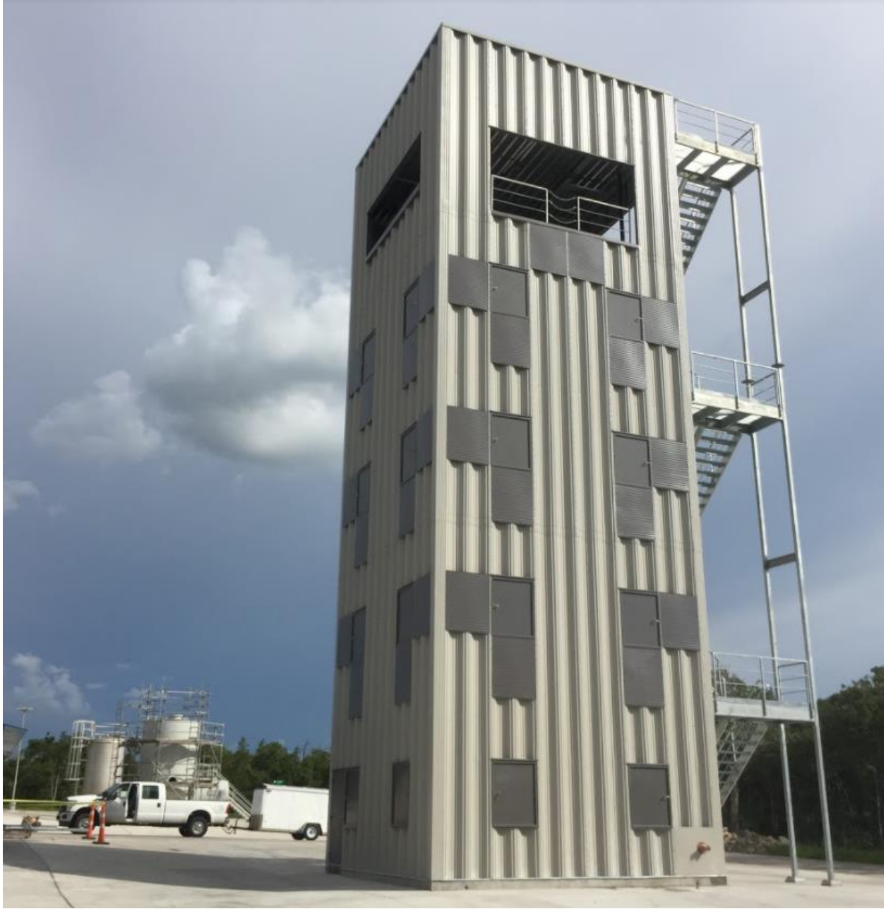
Figure 23: Image of WHP Tower - College Station, TX (WHP, 2015)
