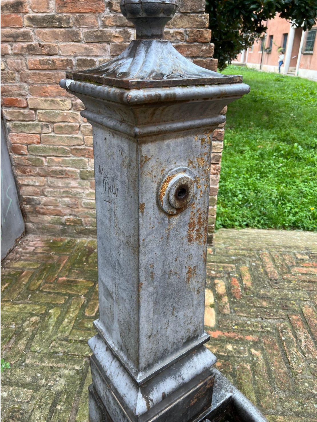
Green Space ID 9: Broken Water Fountain.
