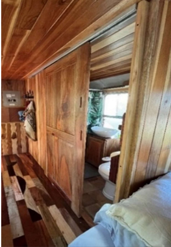
Figure 11. A barn sliding door.
