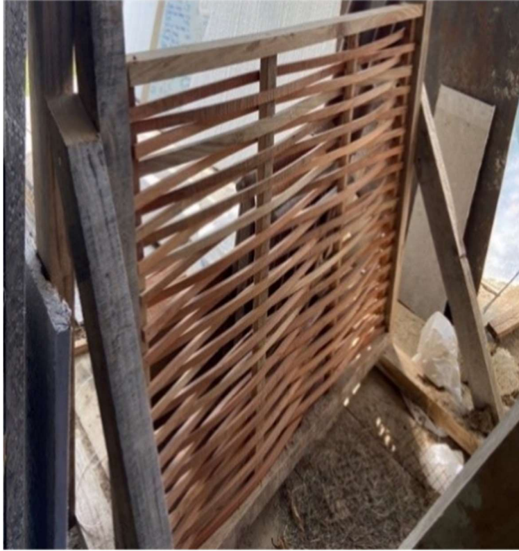
Figure 15. Cedar weave made to apply earthen walls to.
