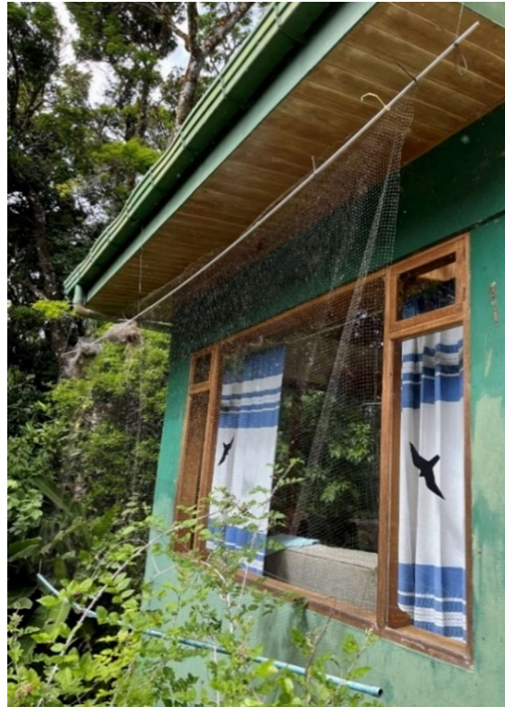
Figure 26. A hanging window mesh.
