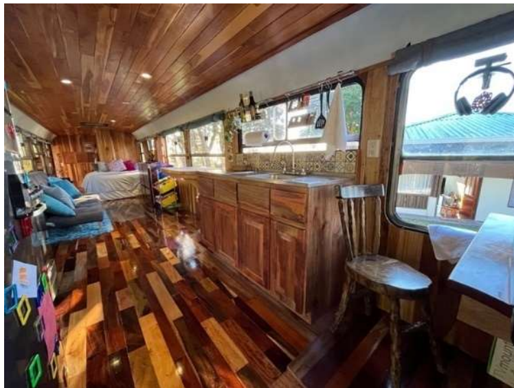
Figure 13. Flooring and furniture made from reclaimed wood and scraps from construction.
