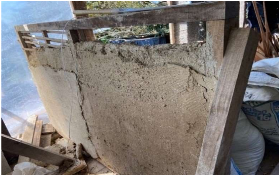
Figure 16. Wattle and daub, applied to the cedar frame.
