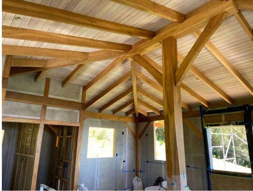
Figure 14. Timber frame home constructed with local teak wood and wattle and daub walls.
