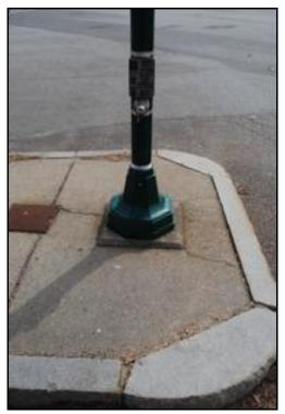
Figure 27: Walking light located on top of an inaccessible median at the intersection of Langley Road and Beacon Street
