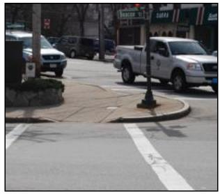
Figure 28: Steep curb cut located at the intersection of Langley Road and Beacon Street
