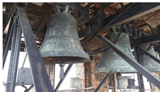
Figure 4.2: Example of A-Frame support
