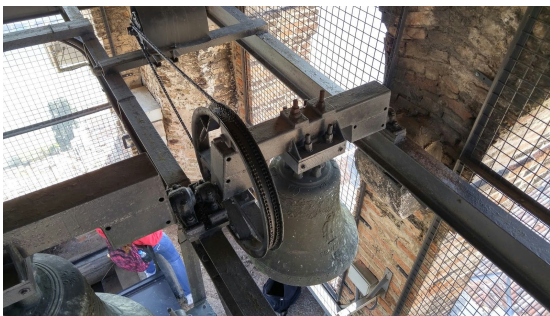
Figure 4.1: Example of H-Frame support
