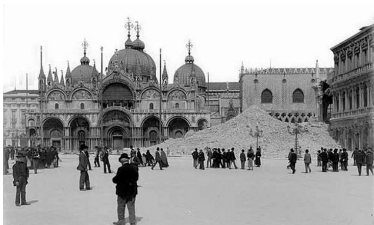
Figure 16: Bell tower San Marco Bell Tower collapse 56
