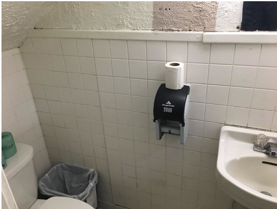
Figure 21. Existing first floor bathroom
