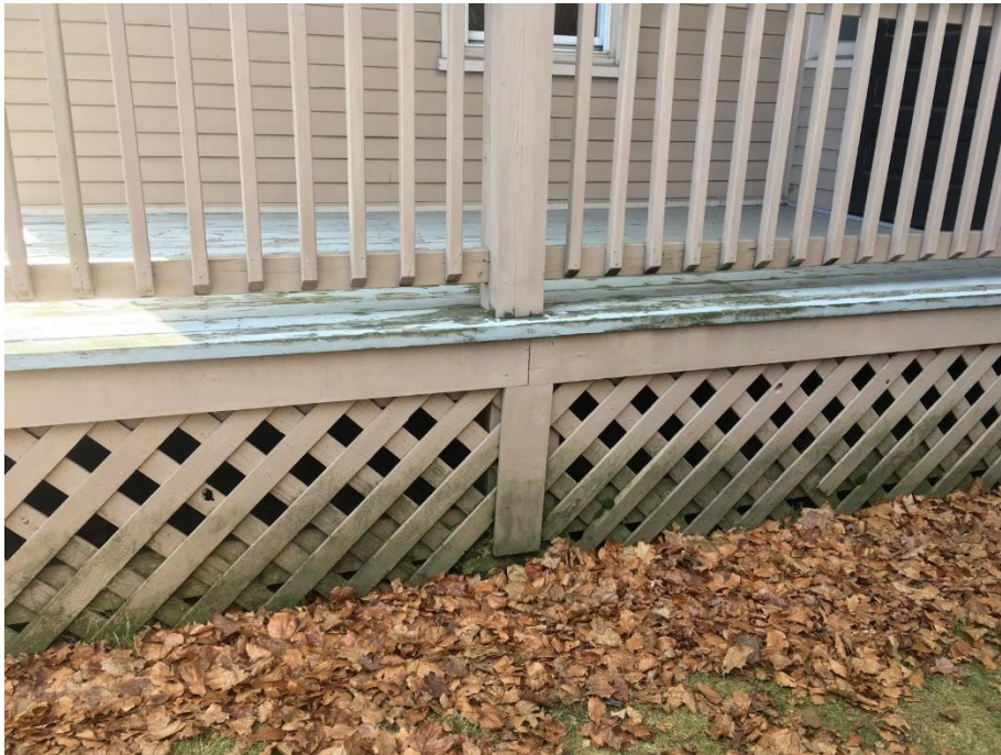
Figure 19. Porch fencing preventing possible window access to Room C
