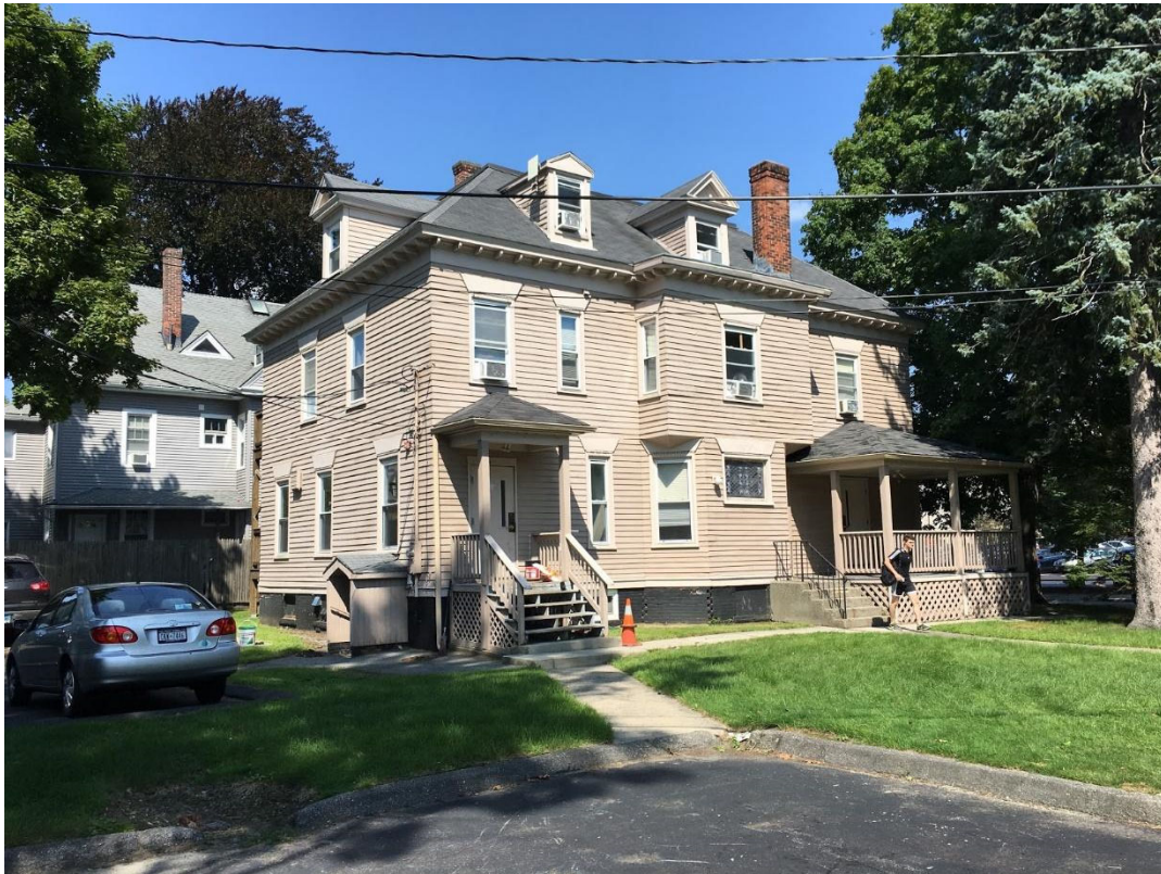
Figure 77. Southwest view of 53 Wachusett Street
