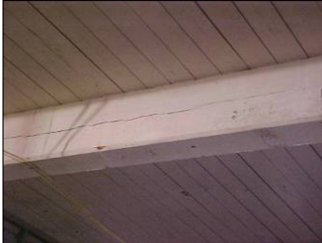
Picture 4: Oak Girder & Southern Yellow Pine Planks
