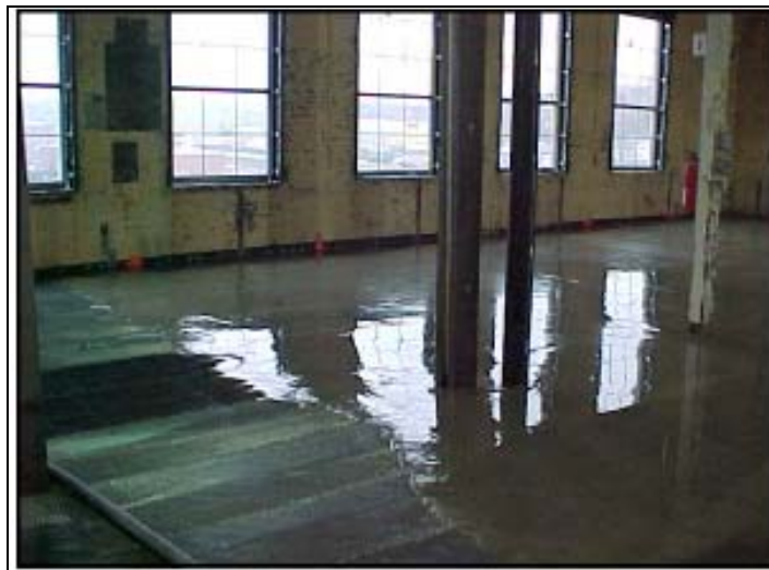
Picture 6: Application of Concrete
