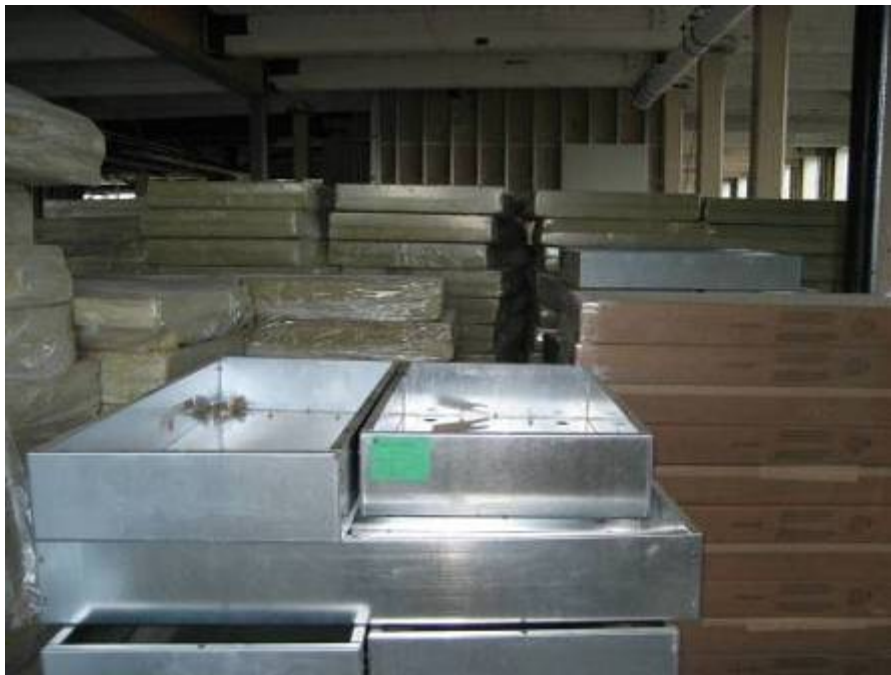
Picture 12: storage on second floor during crack mapping
