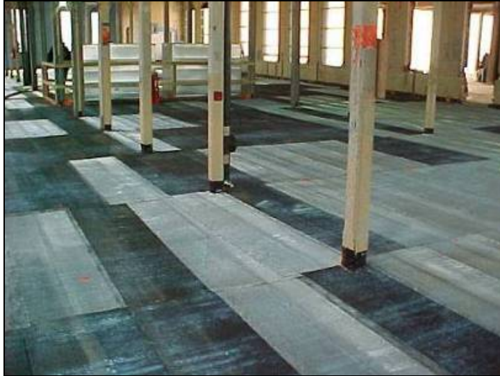
Picture 5: Metal Lath
