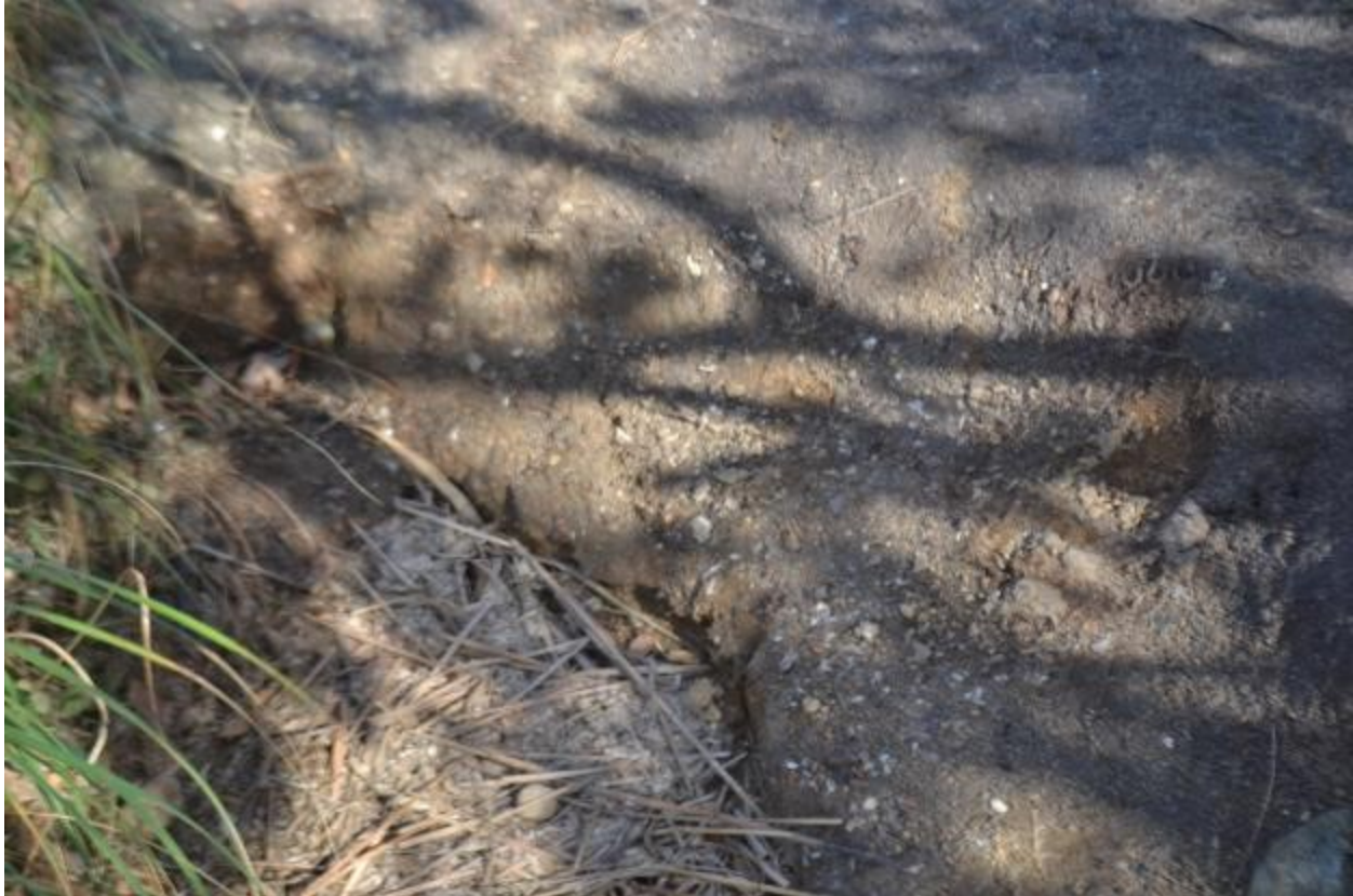
Figure 43: Eroded Path to Dock at 1st Crabbing Location
