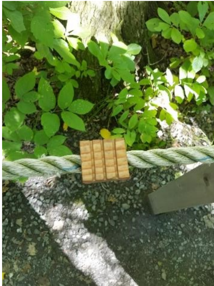
Figure 17: Notification Bead on Post and Rope Guidance System
