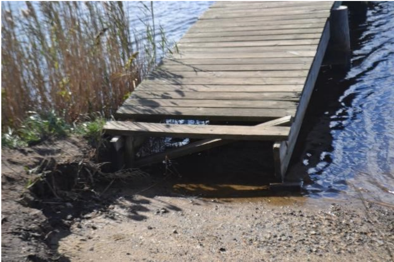
Figure 46: Dock at 1st Crabbing Location
