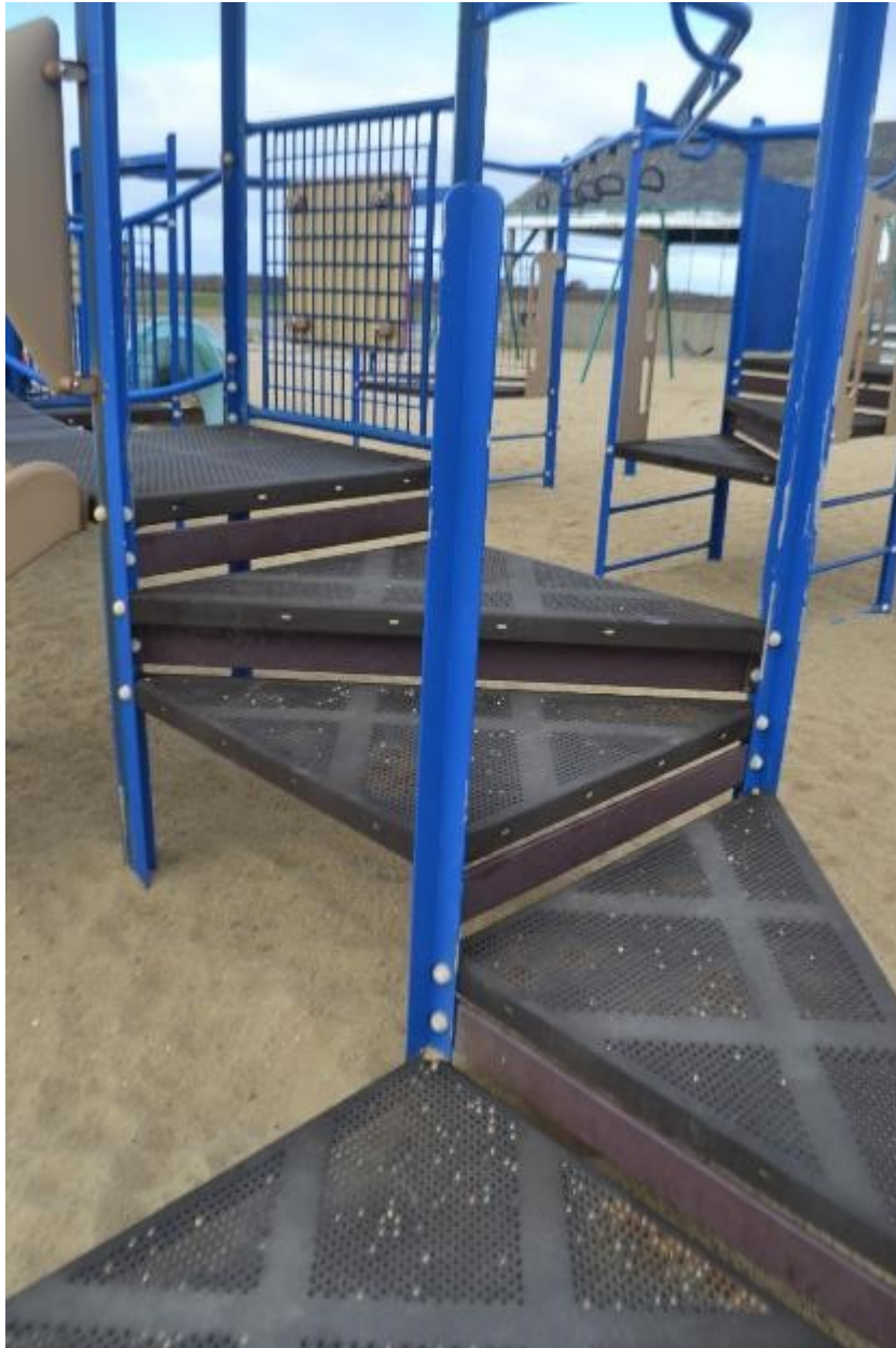
Figure 26: Transfer System on Play Structure at Tom Nevers Playground
