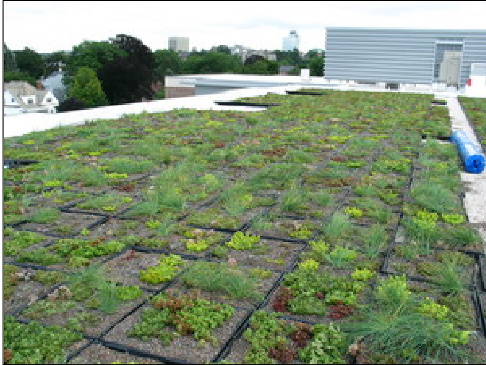
Figure 5: WPI East Hall Green Roof (Martinelle, 2008)
