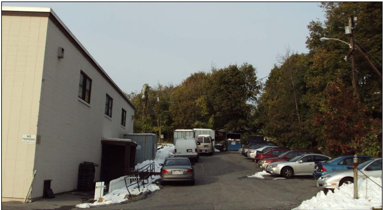
Figure 9: East End of Friendly House Building and Parking Lot
