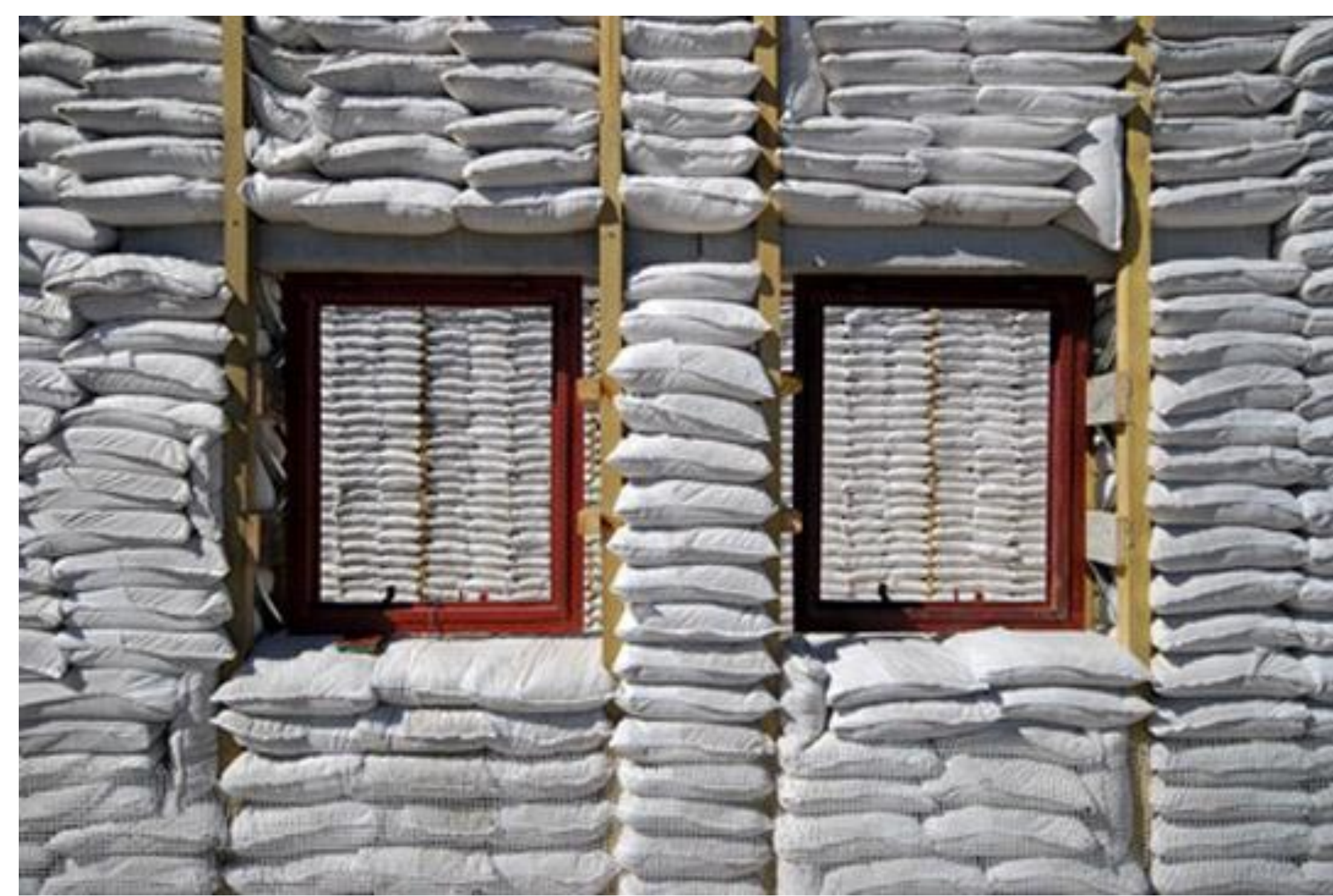
Sandbags will be placed in wall frames to provide weight and stability during hurricanes
