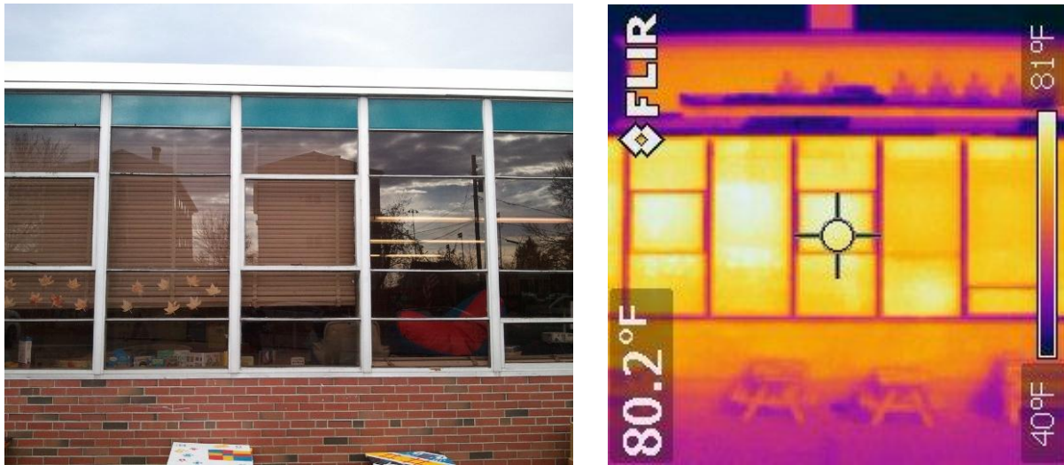
Figure 28. Classroom windows on south side of 1960 building: picture on left, thermal Image on right.
