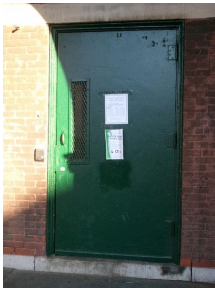
Figure 23. Main door of the 1890 building.
