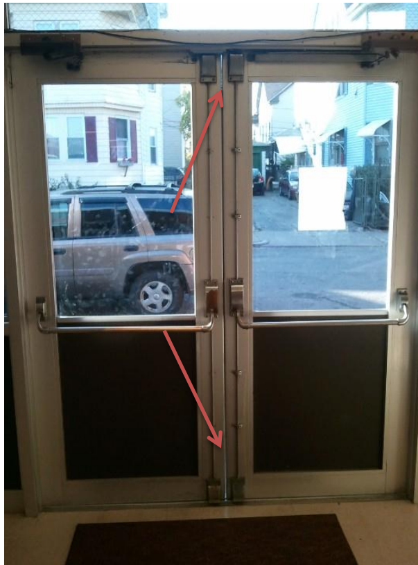
Figure 22. Main doors of the 1960 building (inside).
