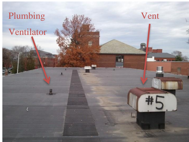
Figure 31. Rooftop of 1960 building East wing.
