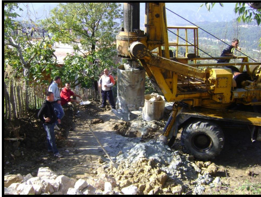
A: Well drilling in the Village of Pellumbas
