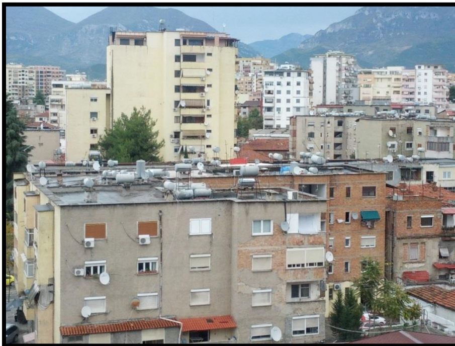
B: Water tanks in a neighborhood in Tirana
