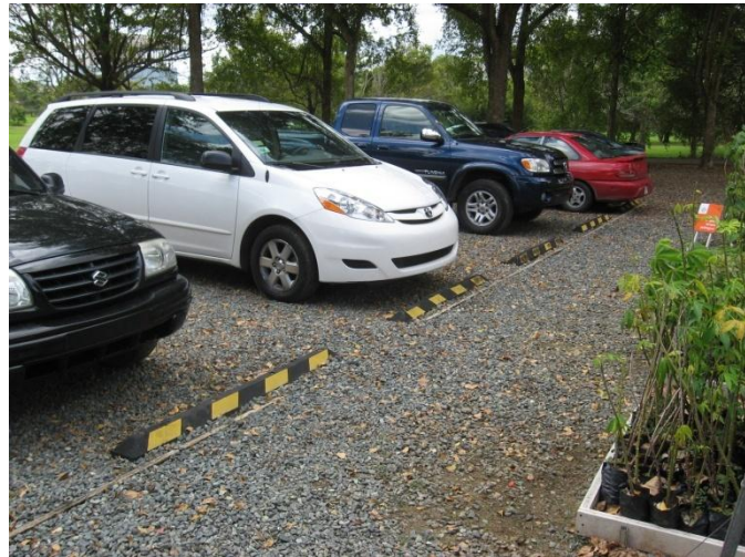
Figure 34: Water Permeable Parking Lot
