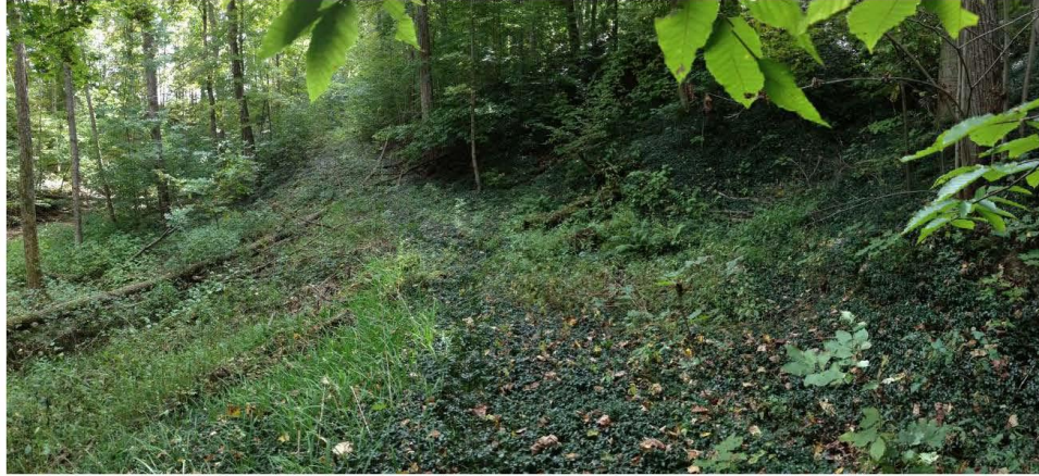
Figure 5: A portion of the proposed ravine trail that experiences frequent drainage issues.
