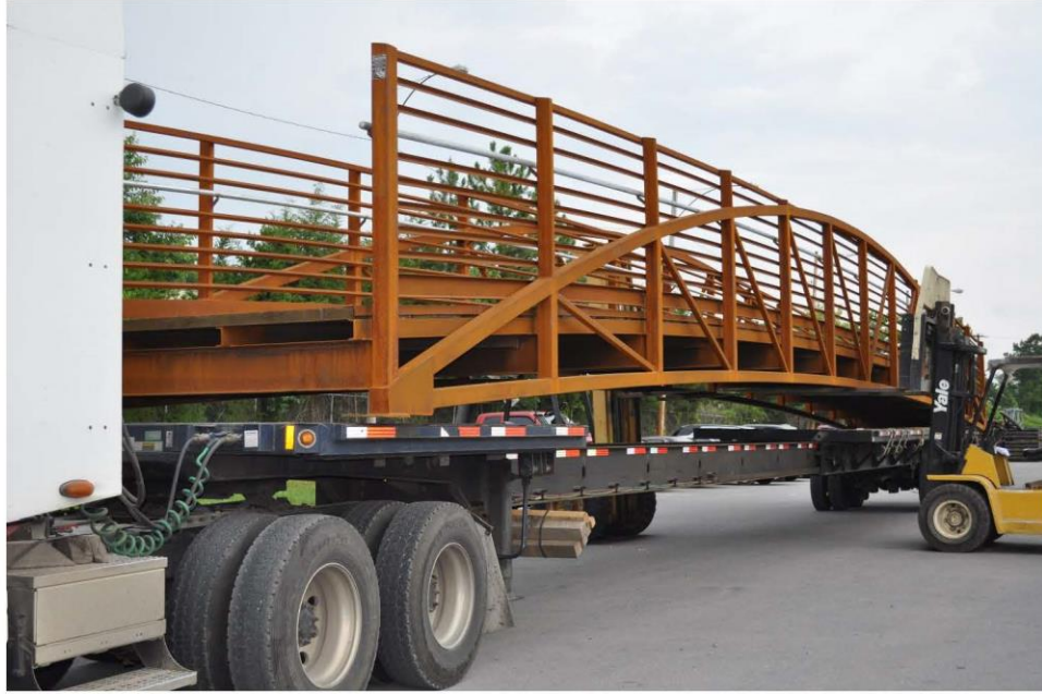
Figure 13: Prefabricated bridge by Pioneer Bridges as it is shipped to the construction site
