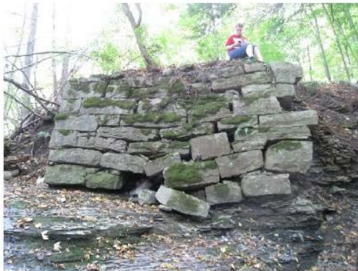
Figure 9: Existing stone abutment
