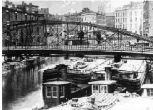
Figure 7: Whipple Truss Bridge circa 1870
