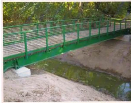
Figure 15: Flatcar pedestrian bridge
