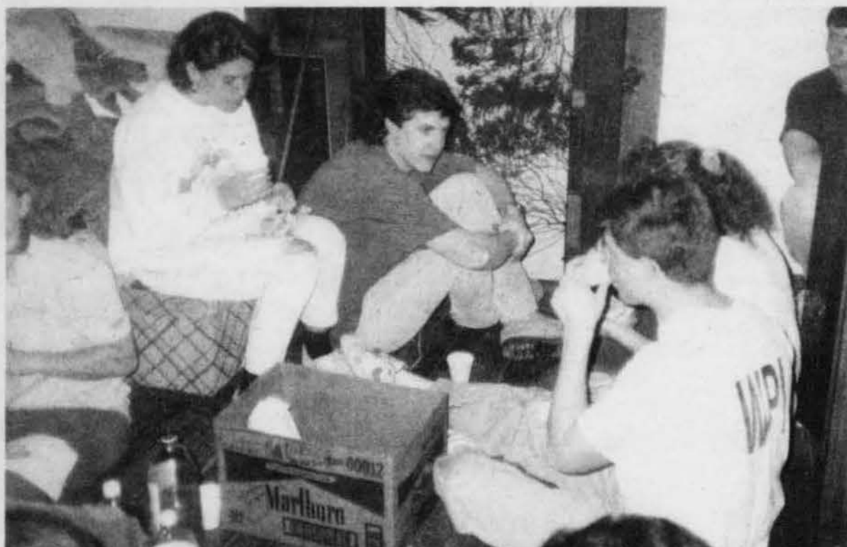
Students take a well-deserved lunch break in between their refurbishment of an apartment for the needy over Spring Break.
