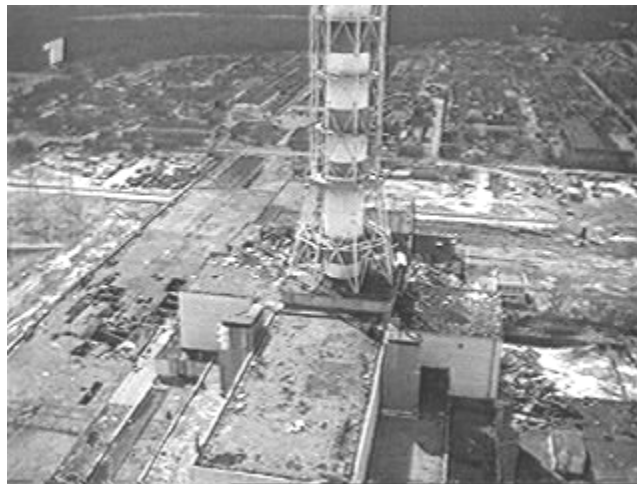
Figure 2: The damage of Reactor No. 4 after explosion
