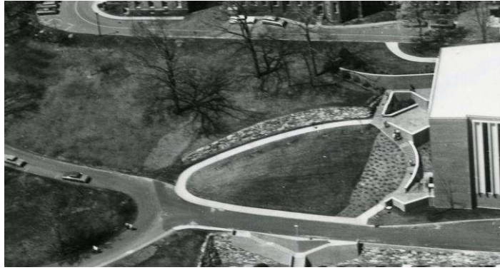
Figure 5: South side first-floor entrance before its removal for the construction of Unity Hall (Library Archives)
