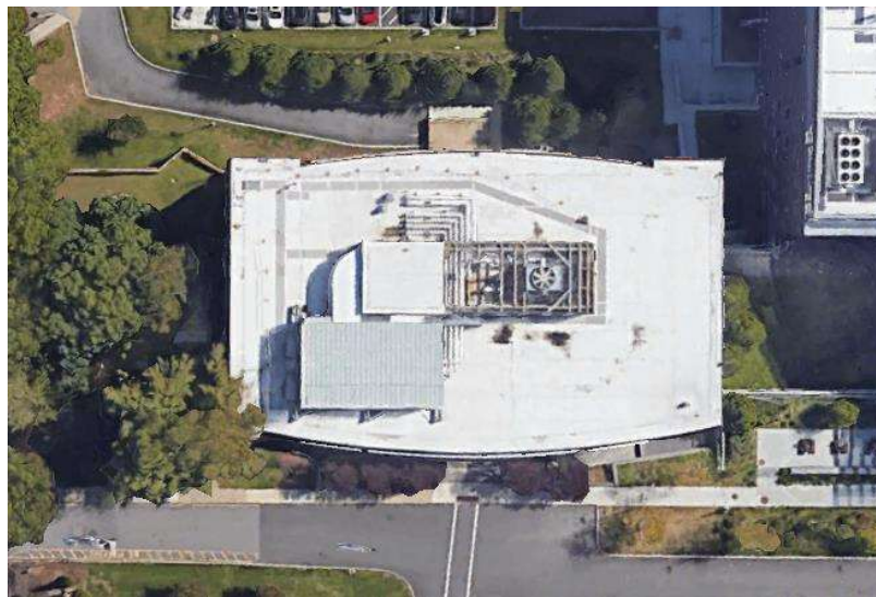
Figure 16: Google Earth screenshot of the library showing the current rooftop HVAC layout (Google Maps).
