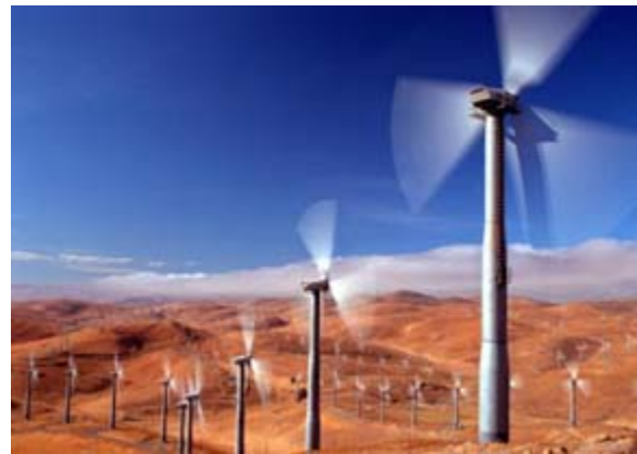
Figure 13: Altamont Pass Wind Farm
