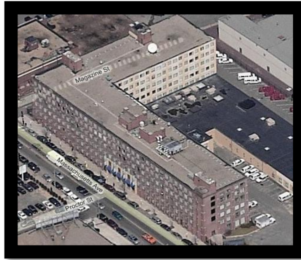
Figure 13: 1010 Mass Ave Aerial View
