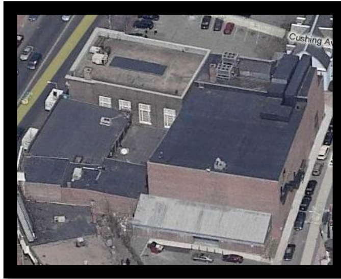
Figure 14: Strand Theater Aerial View
