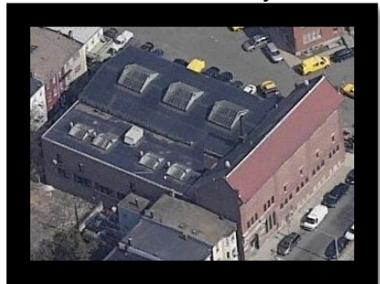
Figure 46: Paris Street Community Center Aerial View
