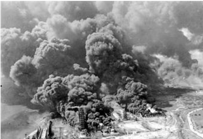
Figure 4: Texas City 1947 Disaster (source: http://www.local1259iaff.org/disaster.html )
