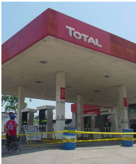
Figure 9: Total gas station
