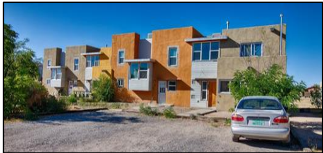
FIGURE 23: THE BACK OF A HOUSING COMPLEX IN TSIKO BUGEH
