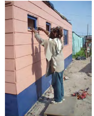
Local Laborer in MWP
