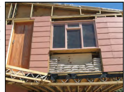
Backpackers Lodge under construction.
