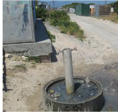
Taps located near toilets can be easily contaminated and aid in the spread of disease
