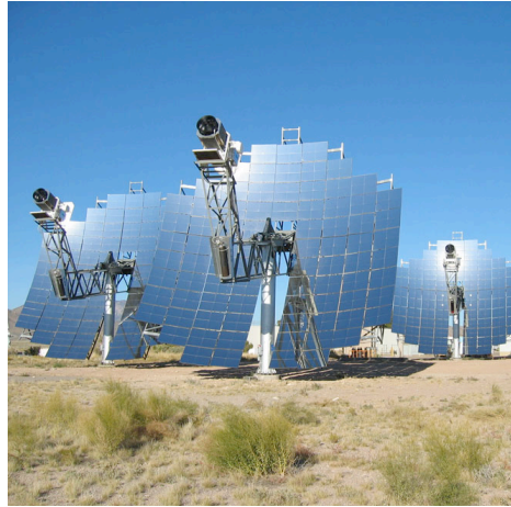
Figure 2-5 SES Solar Dish Stirling System
