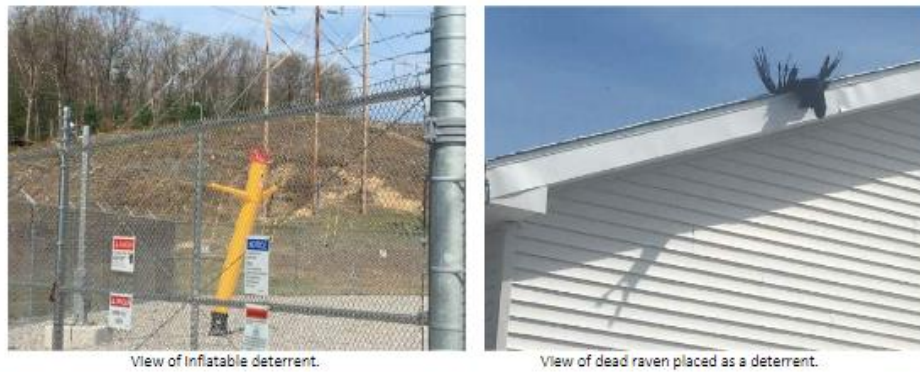
Figure 1: Inflatable deterrent and dead raven deterrent from Rimmon Substation
