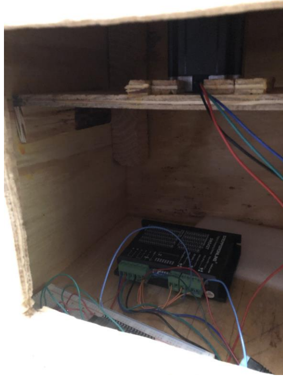
Figure 4: Inside view of the Base Station with the motor and motor driver inside
