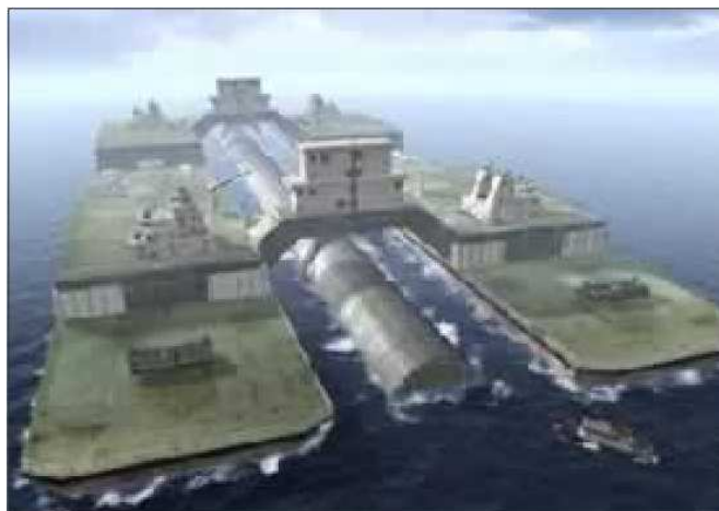
Figure 11: Immersion Pontoon Lowering Tube Section
