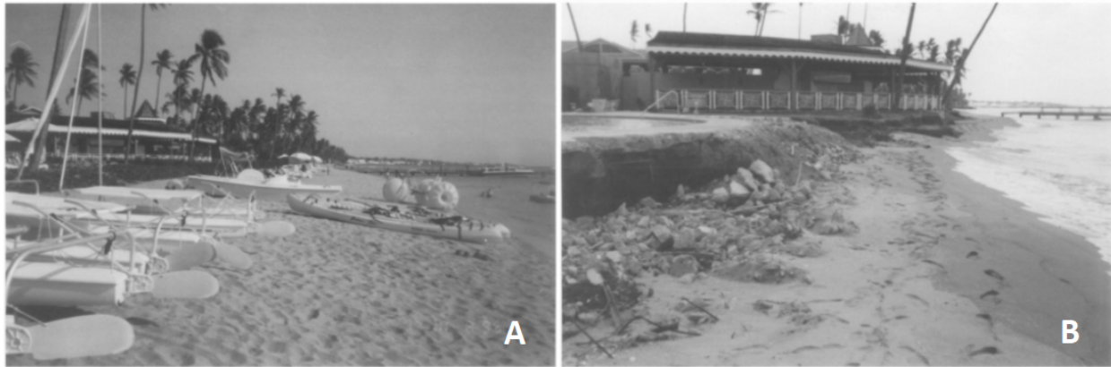
Figure 12. A) Before and B) After Hurricane Luis in Nevis (Cambers, 1997)
