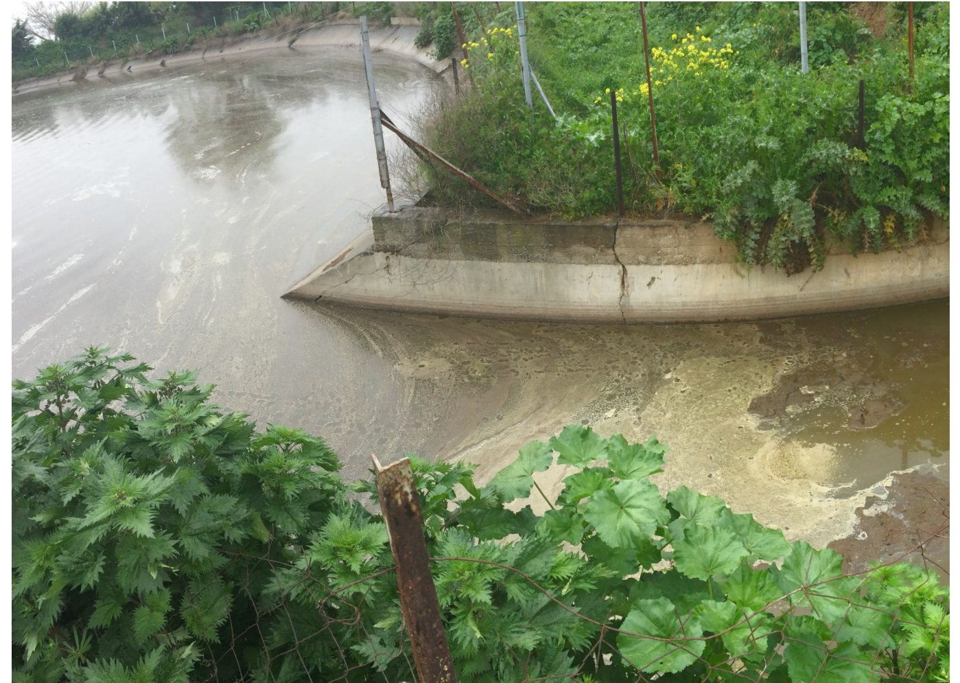
Figure 52: Sludge in the Concrete Lagoon
