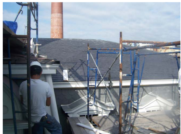
Top Windows and Roof
