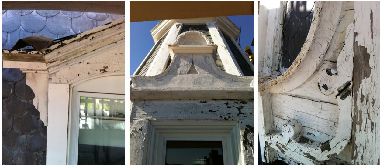
Figure 6. Pre-renovation Window Conditions
