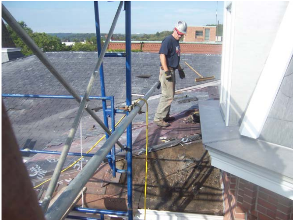
Working on Roofing
