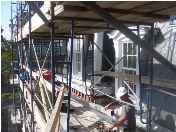
Windows with New Slate
