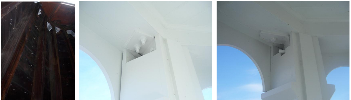
Figure 8. Views of Tower Bracing
