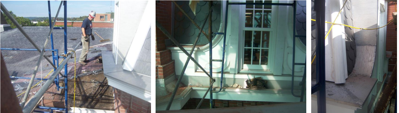
Figure 7. Window Renovation Work
