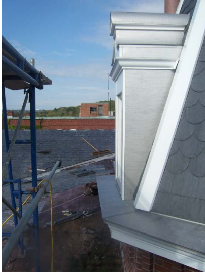
Tower and Roofing
