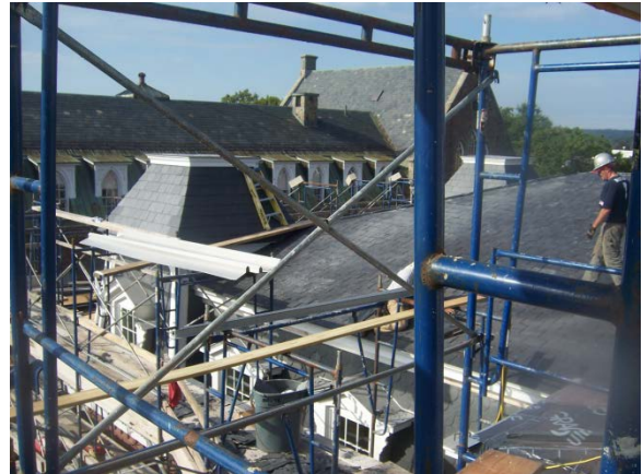
Laying Slate on Roof
