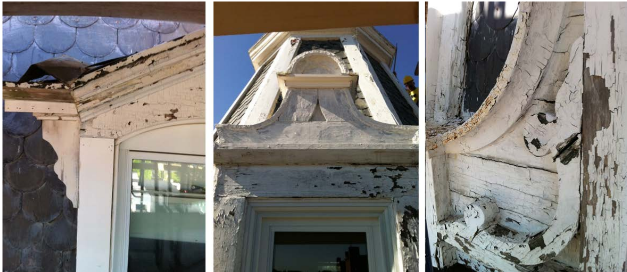
Figure 20: Pre-Renovation Window Conditions
