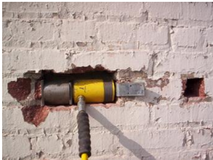
Figure 18. In-place Shear Test
