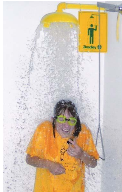
Figure 19. Emergency Wash System (Board of Fire Prevention Regulations, 2010)
