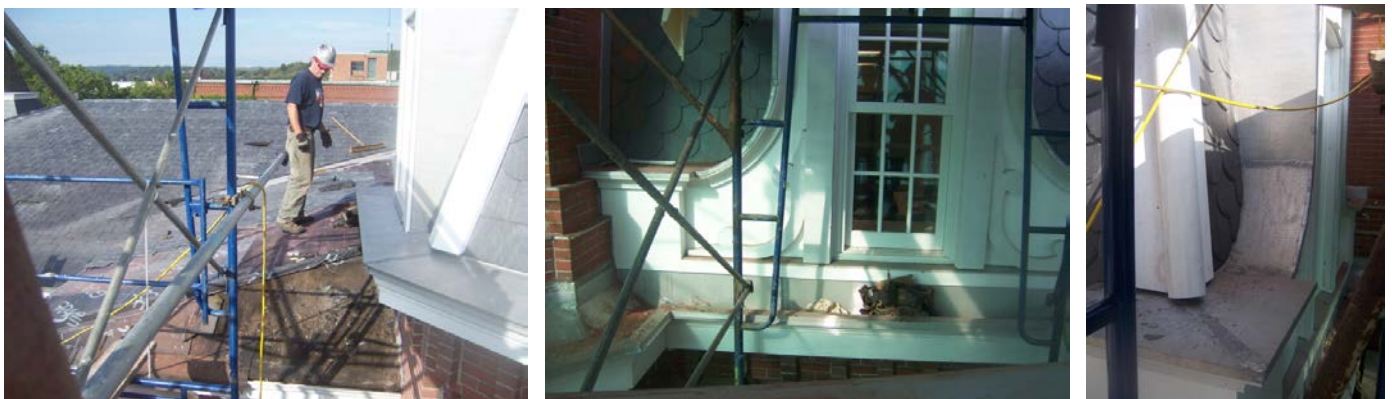
Figure 21: Window Renovation Work
