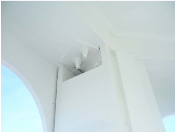
New Exterior Tower Bracket
