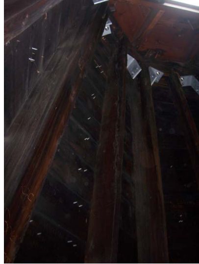
Interior of Tower with New Brackets
