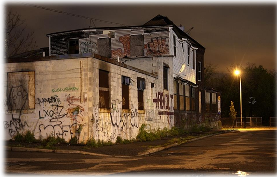
Figure 5: Urban Decay in Worcester, Massachusetts (Donahue, 2009)
