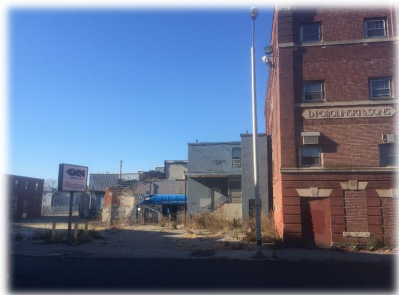
Figure 12: Buildings Along Harding Street in Need of Renovation (photo taken 11/1/14)
