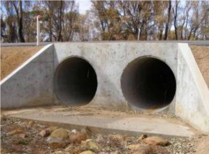
No cracking, piping, or undermining. 4
