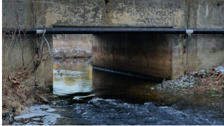
Figure 8: Open-Bottom Box Culvert (Photo: Ryan Bagge, 2014)
