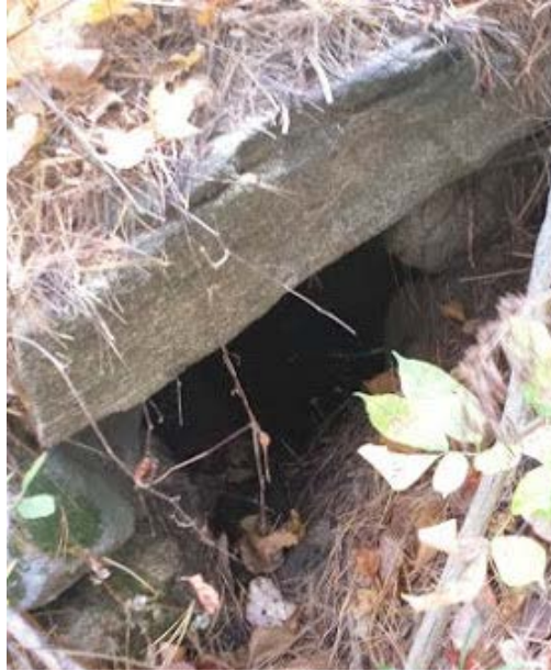
Figure 7: Stone Masonry Embedded Culvert (Photo: Ryan Bagge, 2014)
