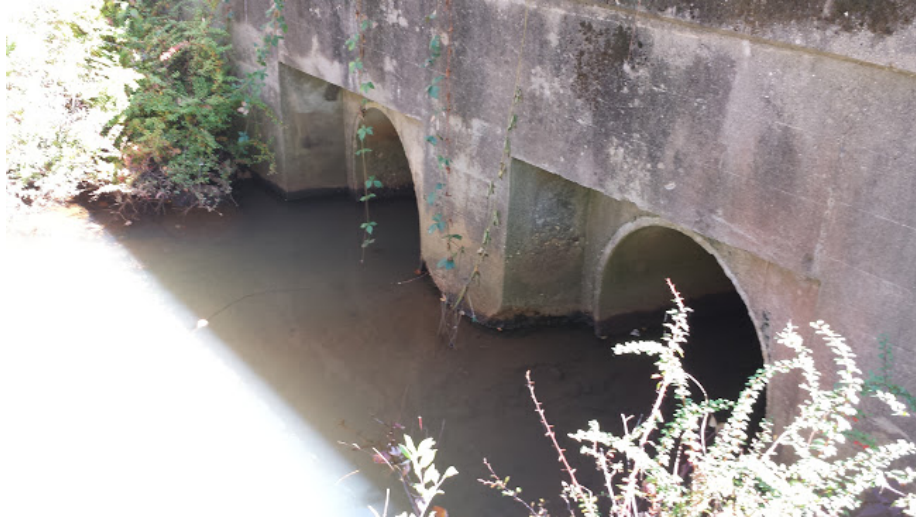
Figure 6: Double-Pipe Culvert (Photo: Ryan Bagge, 2014)
