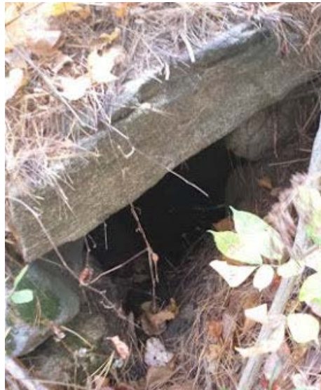
Figure 5 - Stone Masonry Embedded Culvert (Photo: Ryan Bagge, 2014)
