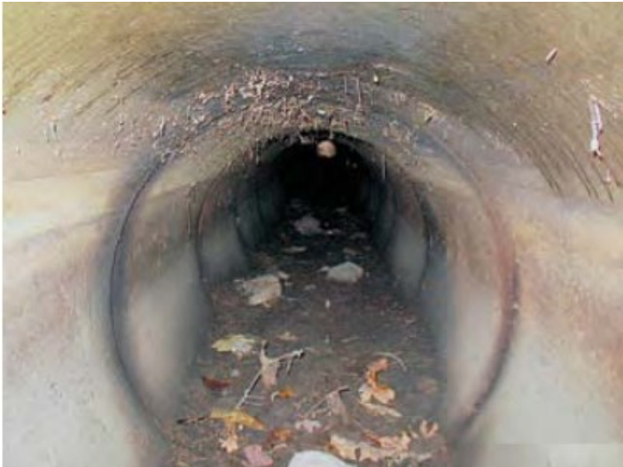
Blockage occupies less than 10% of opening. 1
