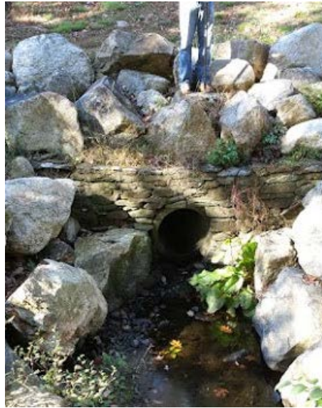
Figure 5: Concrete Pipe Culvert (Photo: Ryan Bagge, 2014)
