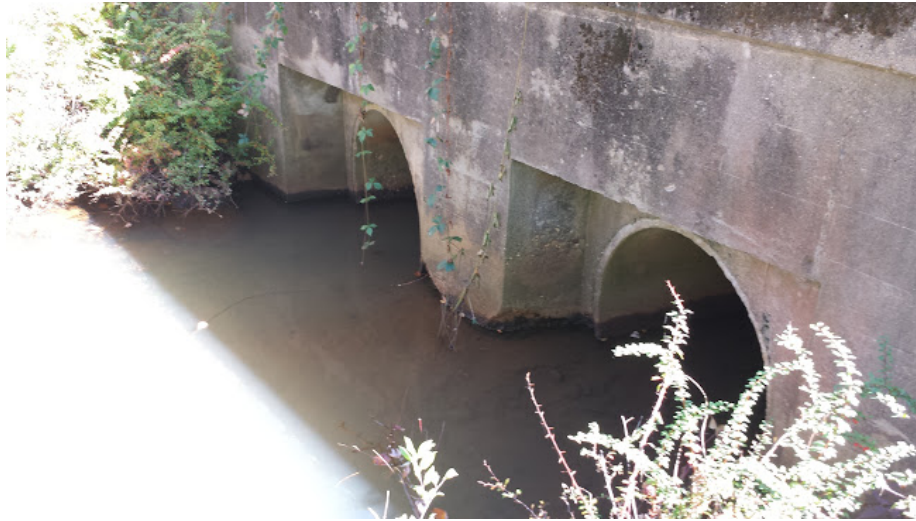
Figure 4 - Double Arch Culvert (Photo: Ryan Bagge, 2014)
