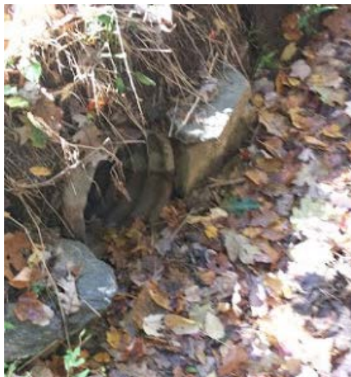
Figure 4: Corrugated Metal Pipe Culvert (Photo: Ryan Bagge, 2014)
