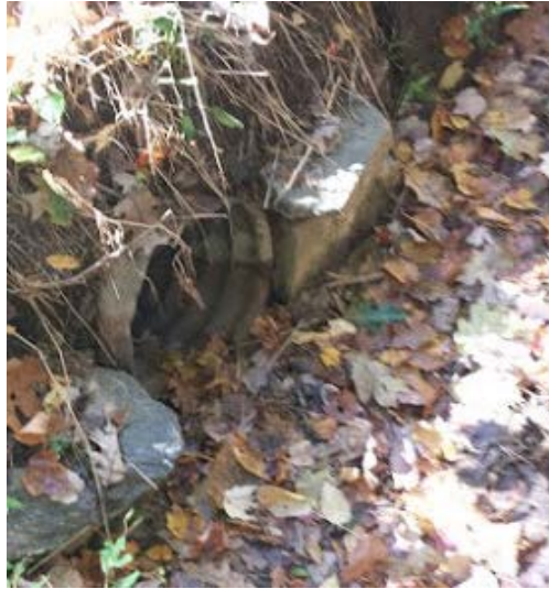
Figure 2 - Corrugated Metal Pipe Culvert (Photo: Ryan Bagge, 2014)
