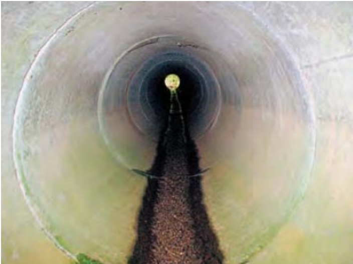
Joints and seams are tight with no openings. 1
