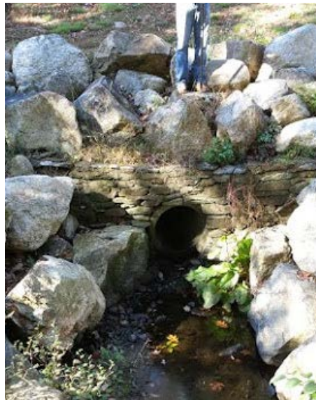
Figure 3 - Concrete Pipe Culvert (Photo: Ryan Bagge, 2014)
