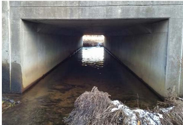
Figure 9: Pre-cast Box Culvert (Photo: Ryan Bagge, 2014)
