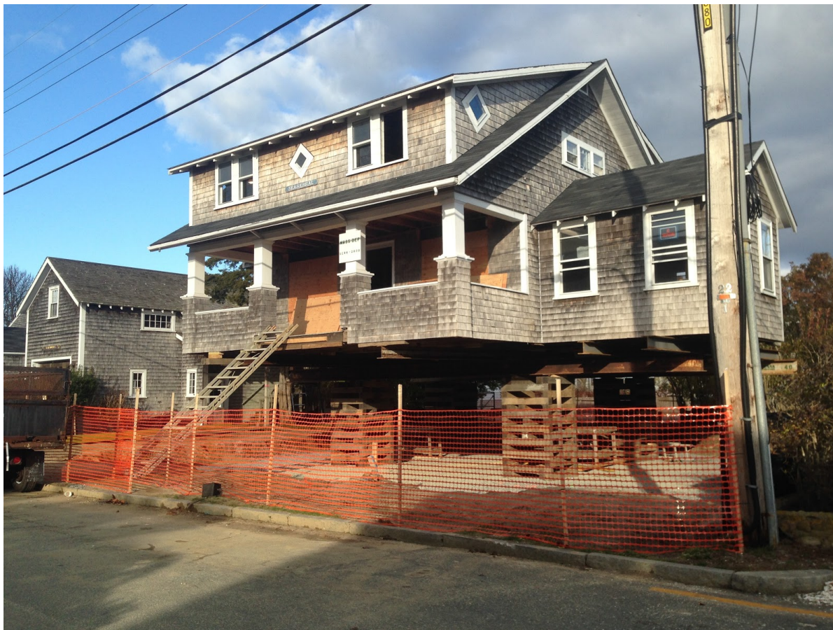
Figure 7: House on Walsh Street, Sitting on Beams and Structural Supports
