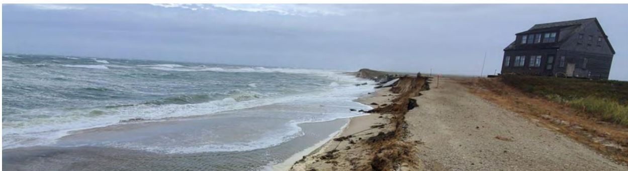
Figure 4: Coastal erosion (NCRAC, 2021).
