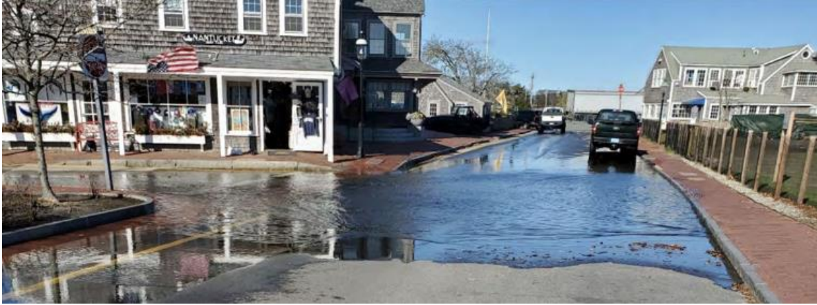
Figure 3: “Sunny day” flooding in downtown (NCRAC, 2021).
