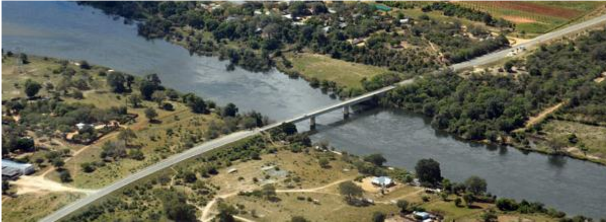
Figure 8: Aerial view of the Divundu Bridge before construction
