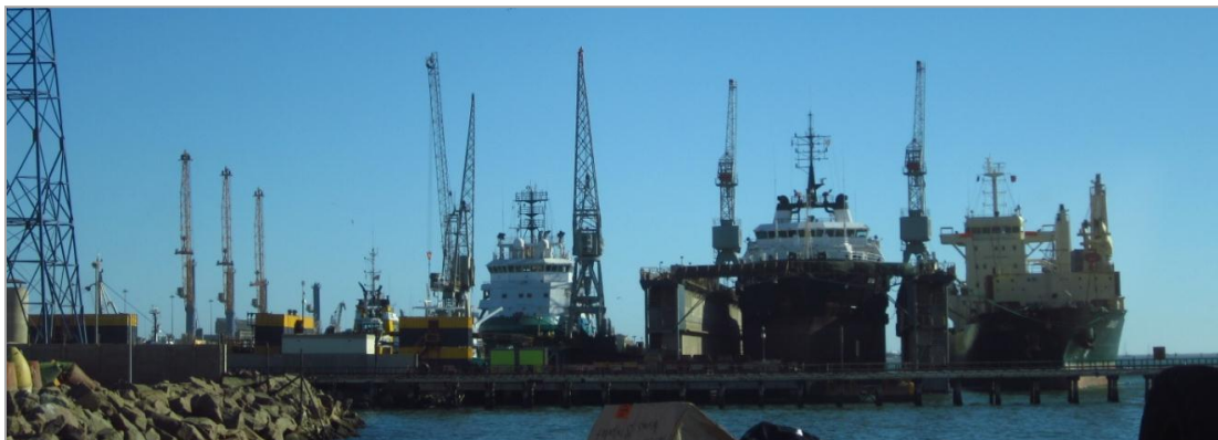
Figure 4: Mobile harbor cranes moving containers from incoming vessels
