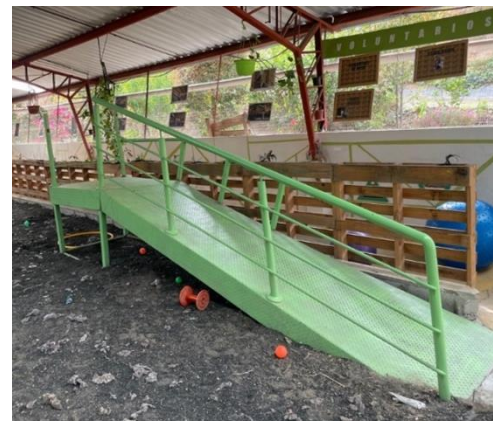
Figure 11. Existing Ramp at Kawallu
