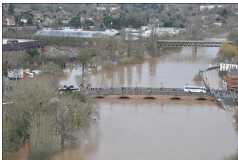
Figure ES1: Depiction of a severe flooding event in Worcester, 2020.
