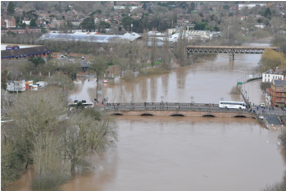
Figure 3: Depiction of a severe flooding event in Worcester, 2020.
