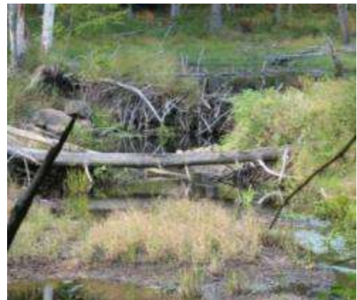
Figure 1: Beaver Activity Upstream of Bridge
