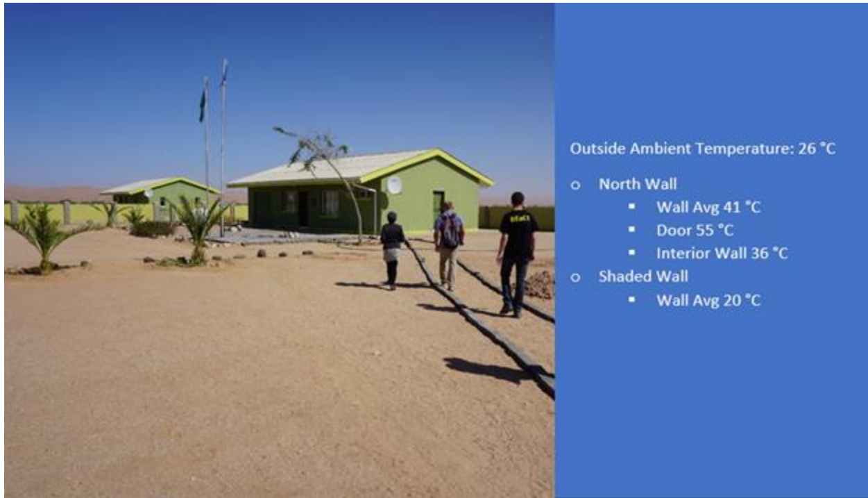
Figure 40. The Topnaar Agricultural Building and the relevant data collected about the building
