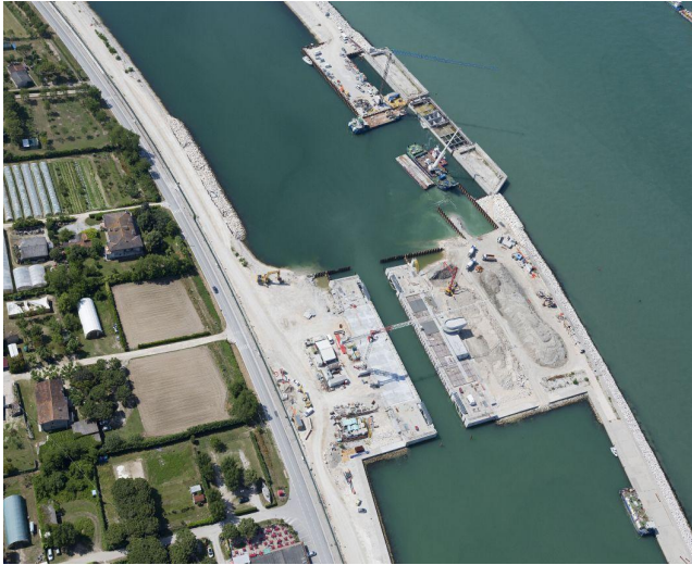
Figure 9. Navigation Lock at Lido Inlet (CVN, 2020)
