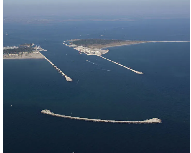
Figure 10. Breakwater in front of Chioggia Inlet (Venice Water Authority, 2020)
