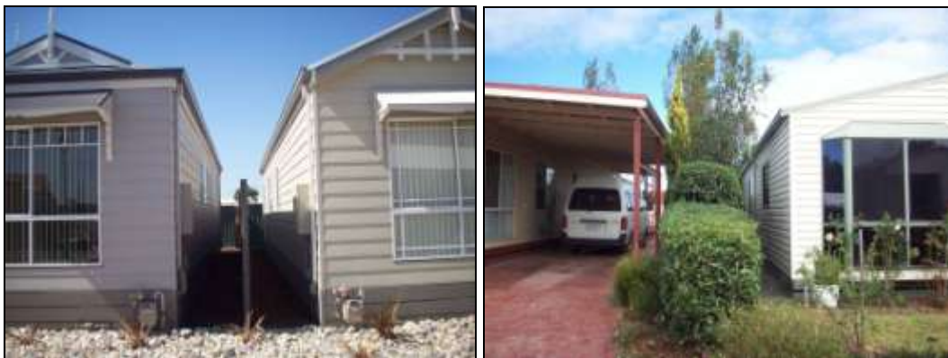
Figure 13 A and B: Obstructed Access Between UMD Structures
