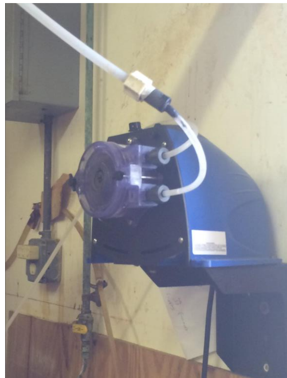
Figure 9: Methanol Pump
