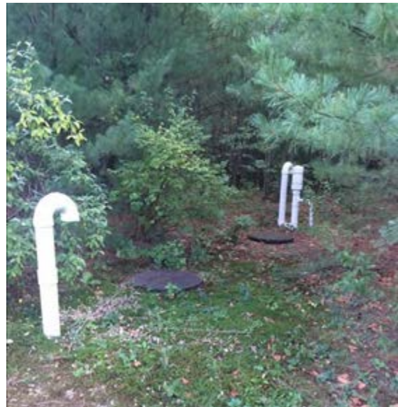
Figure 6: Covers on the Anoxic Tank and FET
