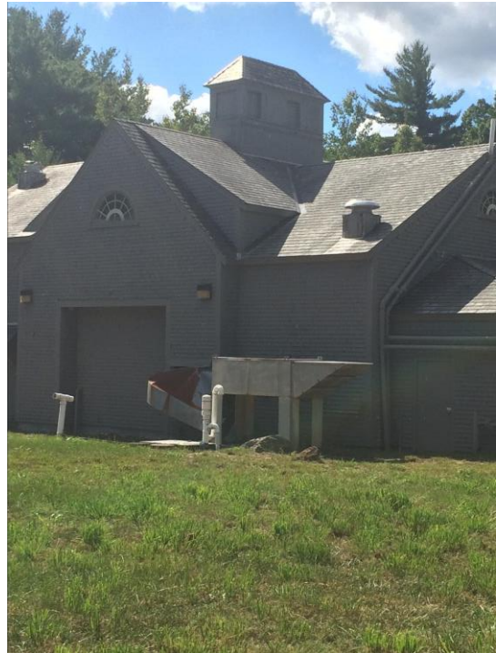
Figure 3: View of the Wastewater Treatment Building
