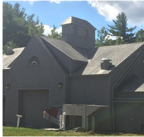
Figure 3: Woodlands Village Wastewater Treatment Building
